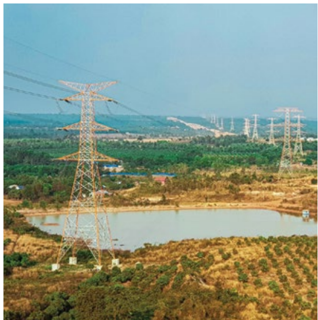
West Phnom Penh – Sihanoukville Project – completed in 2020
