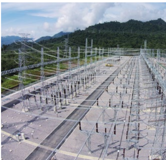
Murum Junction Project – completed in 2015
