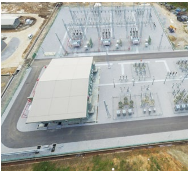
Sakura Ferroalloys Project – completed in 2016
